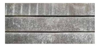
All pre-cast concrete products are susceptible to Lime Bloom which can appear on your concrete sleepers as thin white patches. Lime Bloom is temporary and typically disappears as a result of normal weathering.
